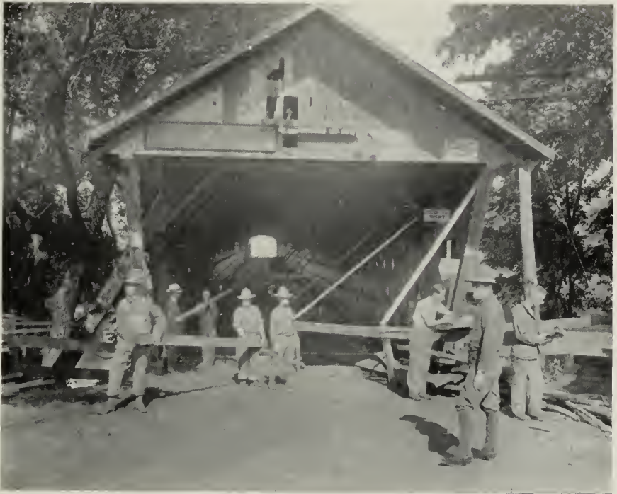
THE LEDYARD BRIDGE RECEIVES A NEW FLOOR
